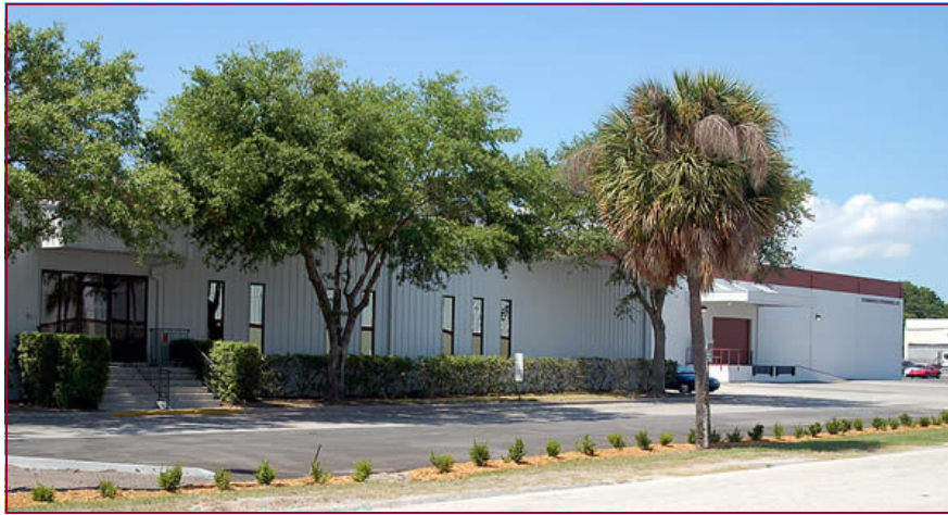
Thermotech's new headquarters and manufacturing facility.
