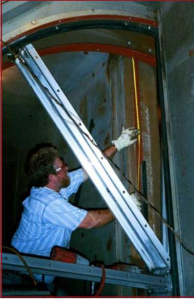
The installation of TR Series wheels can be performed by our trained technicians or by your contractor or staff with our supervision. The casing, when required, is constructed of tubular steel or aluminum and is of a modular design built in either 2 or more sections to provide for easy assembly.
